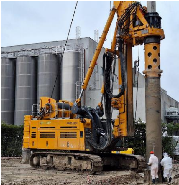
Fig. 5 Drilling machine for D880 mm secant piles.
