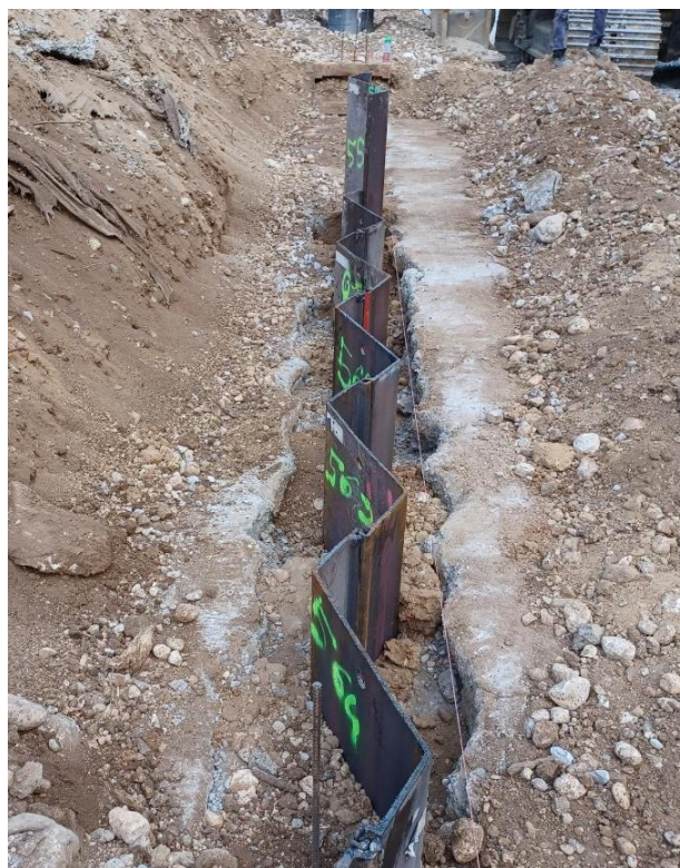
Fig. 4 Relief holes: D600 mm — sheet pile installation.
