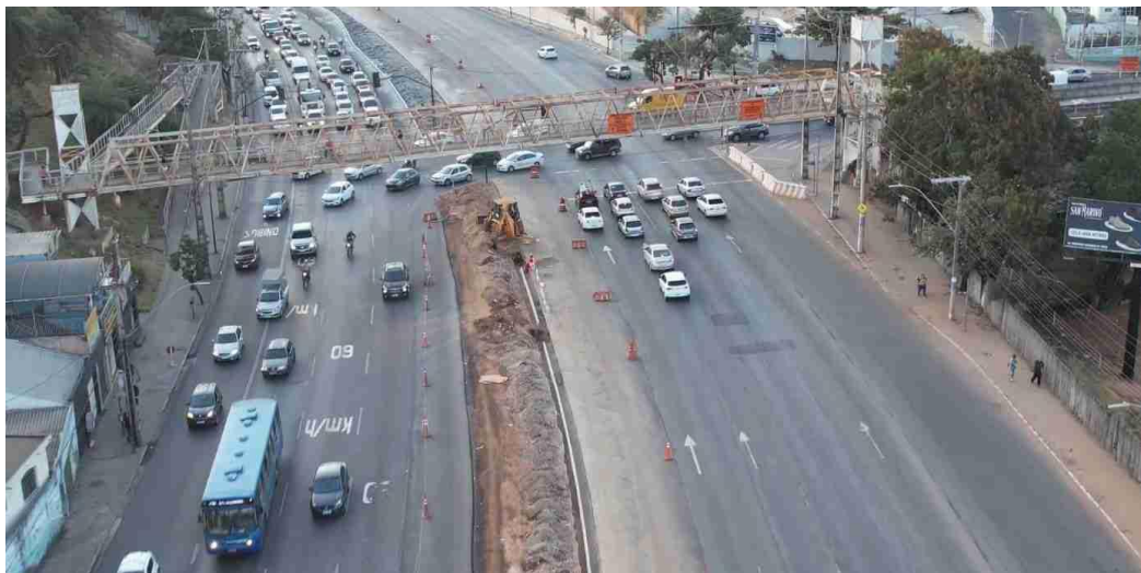
Fig. 11 Monitoring of works on the Waldomiro Lobo Viaduct.
