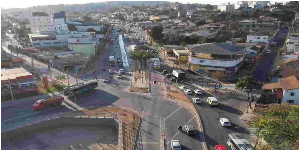
Fig. 4 Monitoring of resurfacing works on the MOVE Vilarinho BRT.
