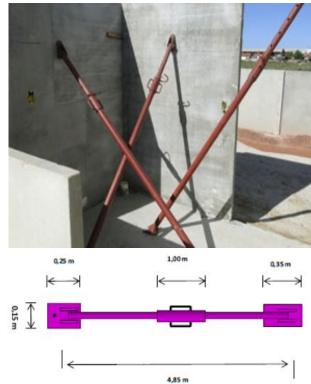
Fig. 2 Shoring and panel locking.
