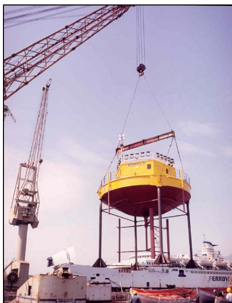
Fig. 9 Turbine at the time of lifting.
