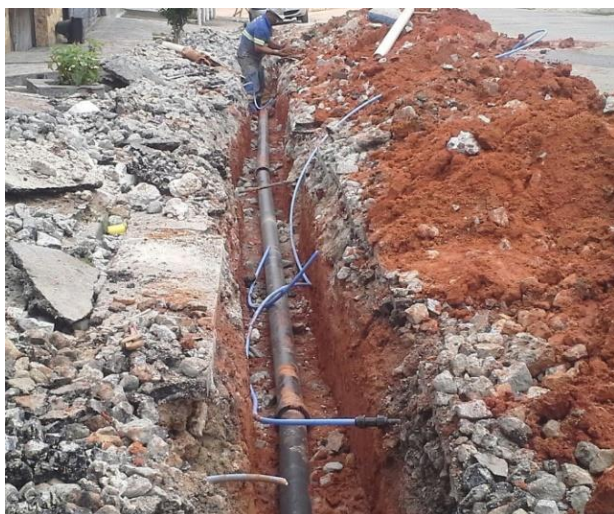
Fig. 8 Distribution network pipes installation.
