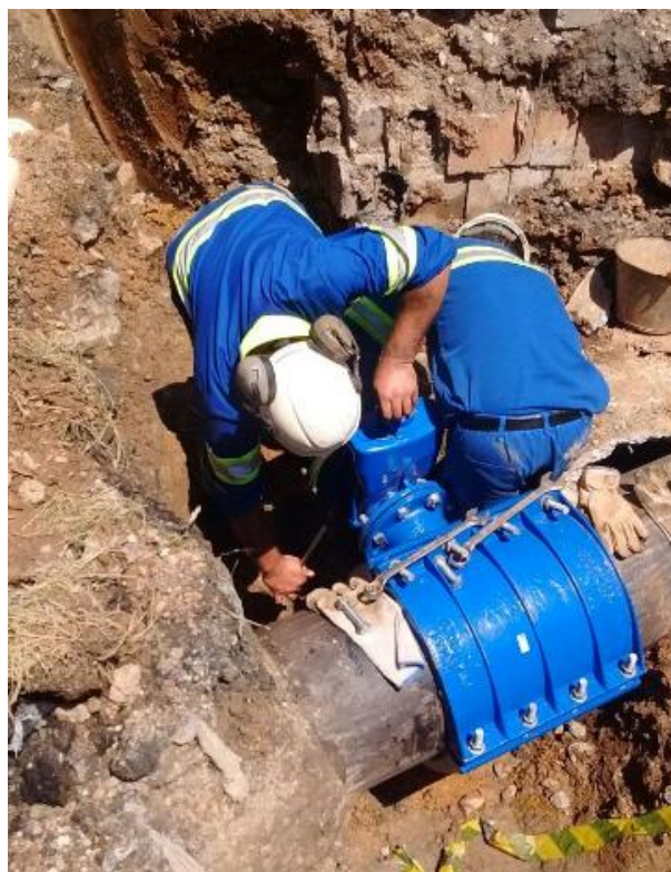
Fig. 9 Installation of shut-off valve.
