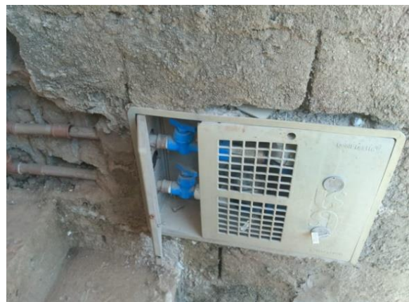
Fig. 10 Installation of hydrometers inside the regularized water connection box.
