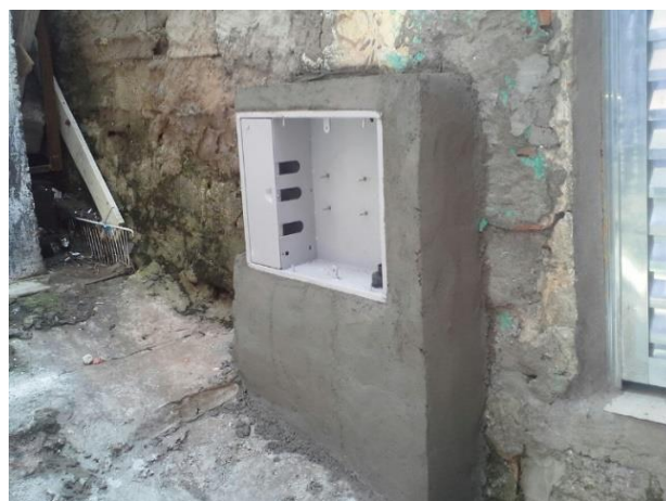
Fig. 7 Installation of regularized water connection box.
