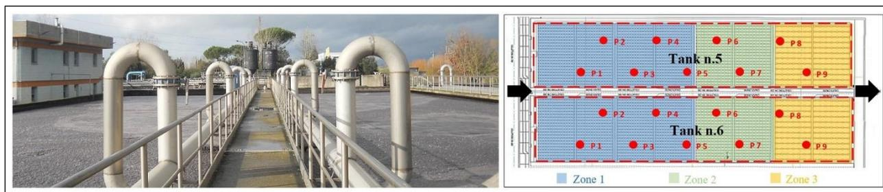
Fig. 2 Cuoiodepur WRRF oxidation tanks (left); scheme of measuring points and the three different diffuser density zones in the two tanks (right).
