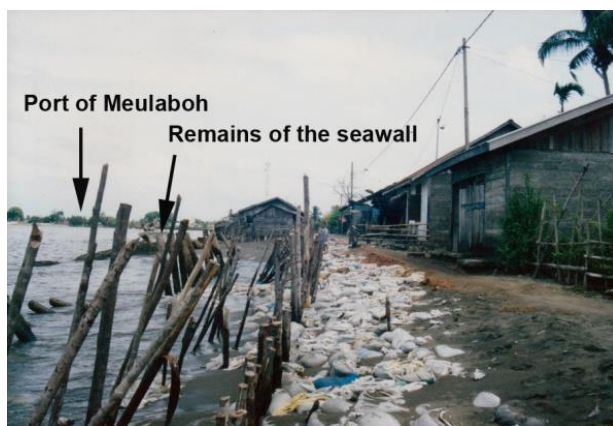
Fig. 4 Coastline erosion at Padang Seurahet in August 2002. Coastal erosion was damaged seawalls, residential roads and houses. (Photograph: WB Setyawan, Agustus 2002).
