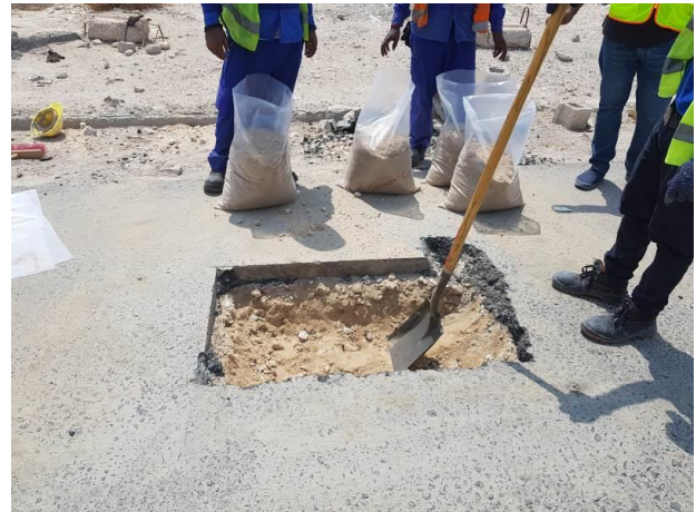
Fig. 4 Exposed subbase and sampling of the control unbound materials.
