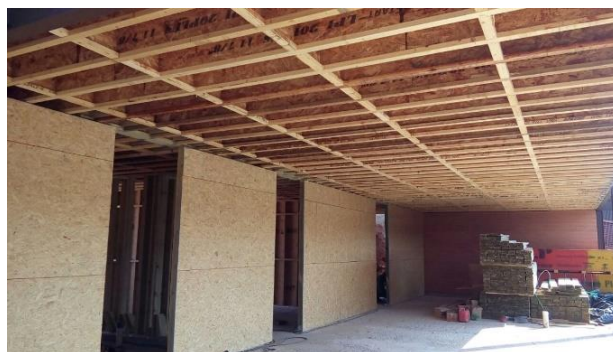
Fig. 4 Casa Terra wood frame walls and slab.
