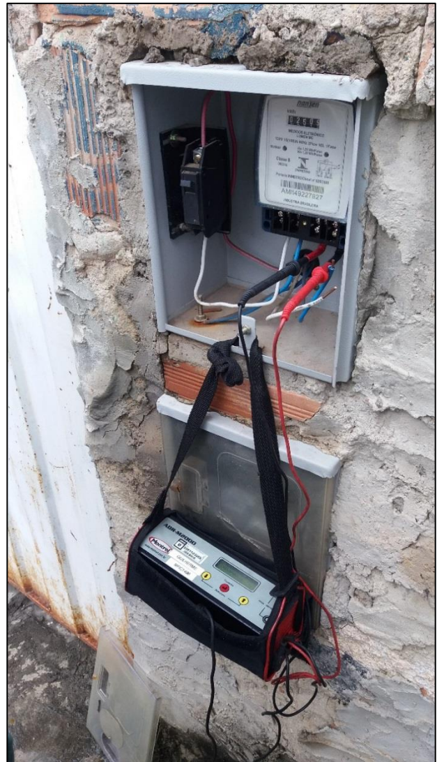
Fig. 1 Inspection in Consumer Unit. Source: Judicial Inspection performed by Pedro Alberto Brasil Vieira dos Santos Process n.º: 0024.13.314.051-7 – October 2010).
