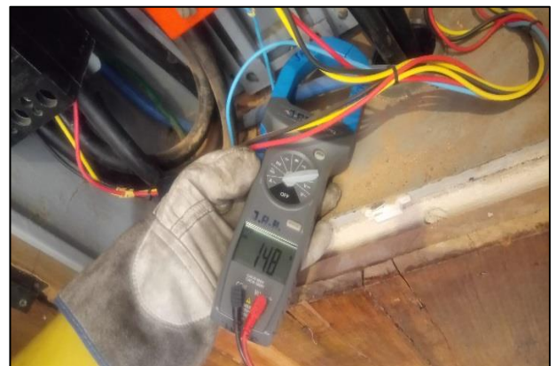
Fig. 2 Inspection in Consumer Unit. Source: Judicial Inspection performed by Pedro Alberto Brasil Vieira dos Santos (Process n.º: 0024.14.093.026-4 – July 2017).
