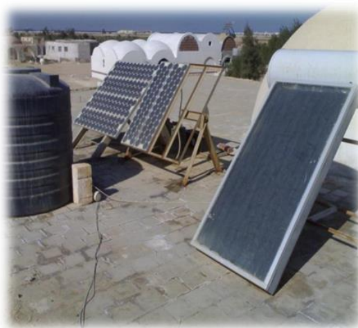
Figure 7 Solar Energy Systems (PV and Solar Water Heater) Installed on the Roof Top of the Common Room in the New Basaisa Community (1996).
