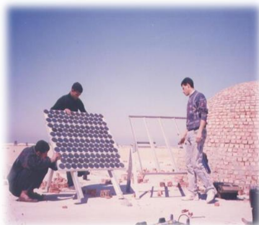
Figure 5 Installation of a Solar System on the Roof Top of a House in the New Basaisa Community As Part of Community-Based Training and Local Capacity Building.
