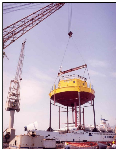
Fig. 9 Turbine at the time of lifting.
