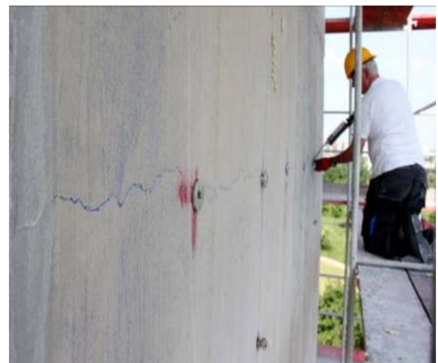
Fig. 6 Horizontal scratch, thickness of about 0.5 mm.
