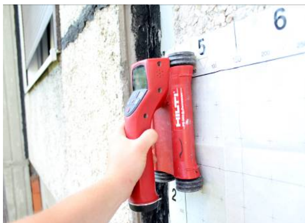
Fig. 14 Scanning the reinforcement with the Ferrosan PS200 device.
