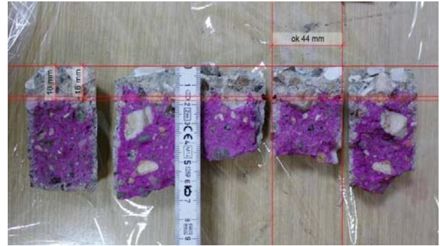
Fig. 10 Visualized analysis of the carbonation range of the external layer's concrete.
