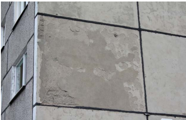
Fig. 7 Degraded cardboard layer.
