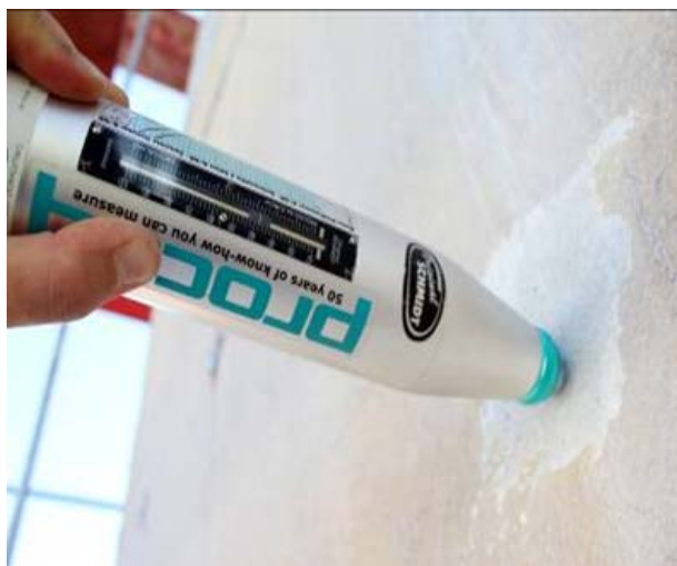
Fig. 13 Measurement of the L rebound number on a smooth surface of an end wall.
