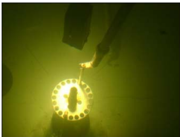
Fig. 14 Removal of old sources from the open basket.
