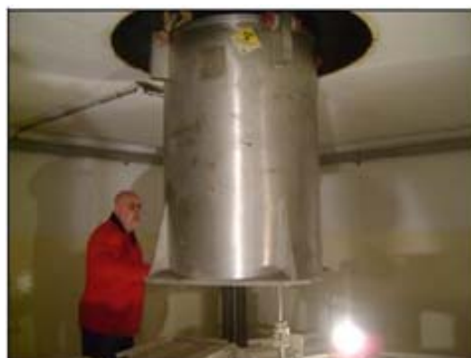
Fig. 5 Removal of SV-68 container.
