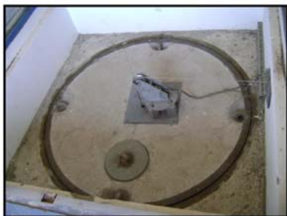
Fig. 23 Top view on the roof plug after removal of temporary pool.
