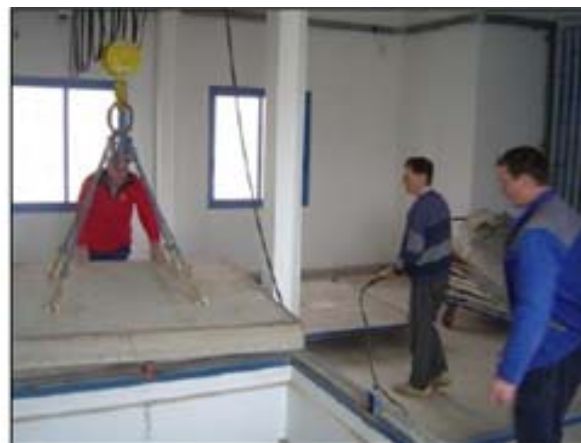
Fig. 24 Roof cover and plug reinstalling.
