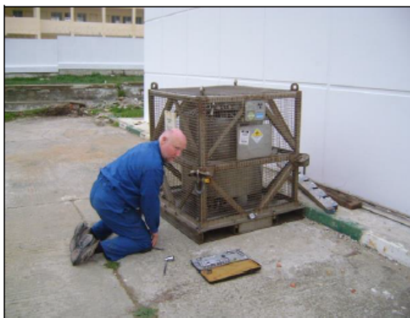
Fig. 17 B(U) Type Package dismantling.
